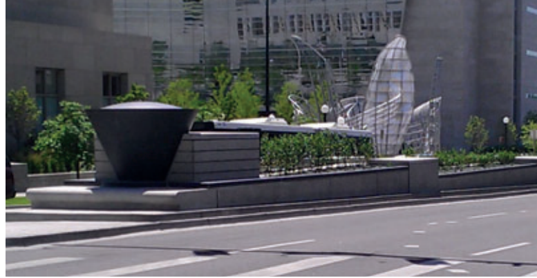
1f -- Median precast elements by StoneBilt Concepts are a key component along Colfax Avenue outside Denver's new Justice Center.
