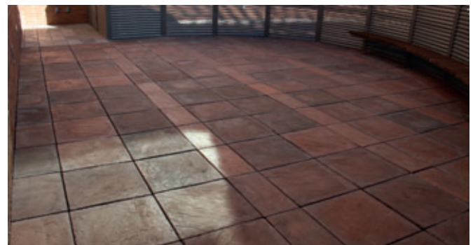
1b -- Sandstone textured pedestal pavers – Childrens Hospital – Aurora, Colorado
