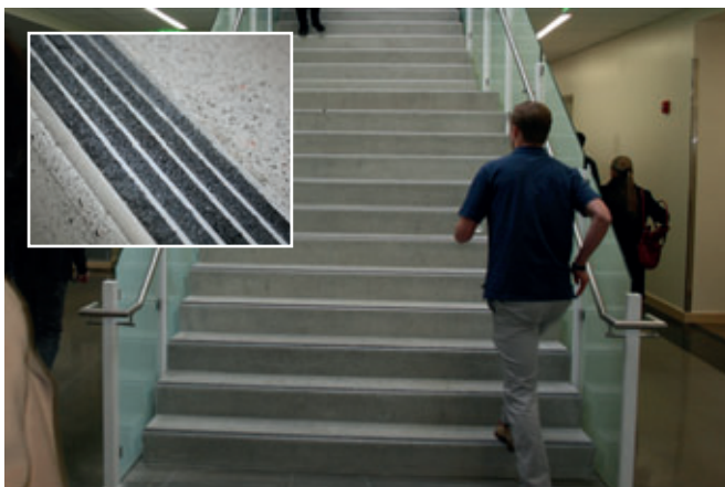
1c -- Custom stair riser and tread components for Colorado Academy High School.
