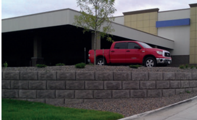
1e -- Lock+Load™ retaining wall for retail store in Centennial, Colorado.
